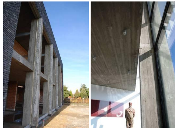
Fig. 18.2. concrete structure on a grid (left); Fig. 18.3. detail of structure (right).
